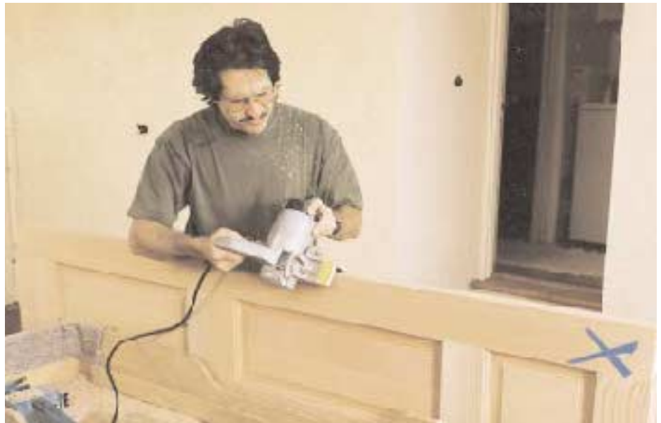
Figure 4. To avoid confusion when beveling the stiles, always work with the X facing toward the work bench. Make several passes with the plane, taking a small amount of material each time and holding the guide firmly against the face of the door to avoid a wavy reveal (top). The last step is to tip the plane to ease the edges (above).
