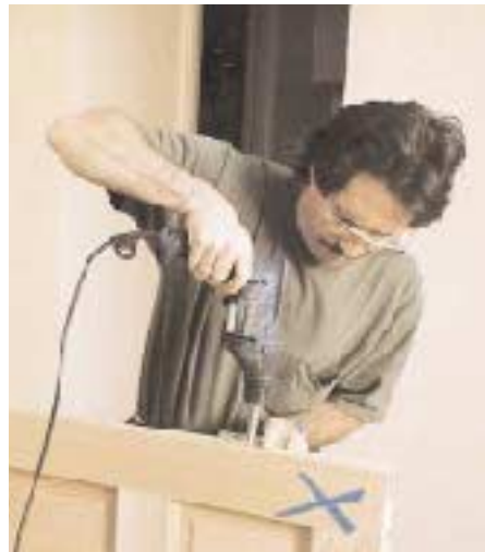
Figure 5. To mount hinges quickly and accurately, the author attaches a template over the hinge marks (top), then uses a router to cut the mortise (above left). Predrilled holes and a Vix bit speed the driving of the hinge screws (above right).
