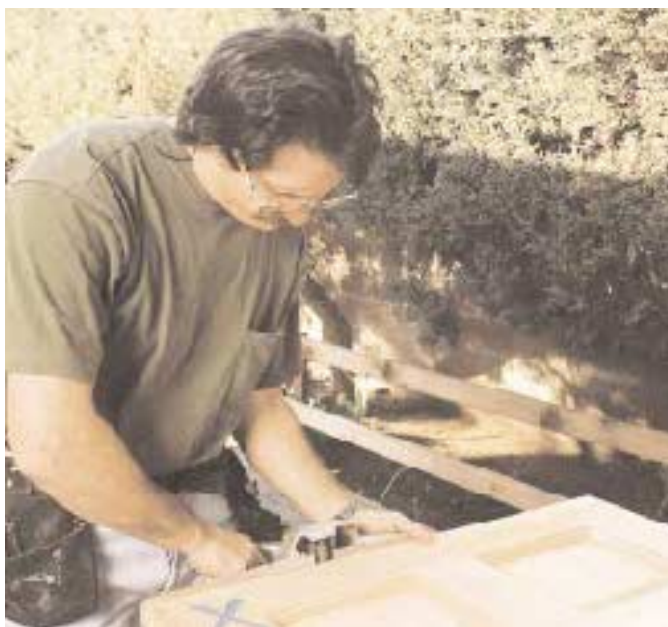
Figure 3. To ensure an even reveal at the top of the door, cut close to the scribe line with a circular saw, but finish the job with a power plane. To avoid tearout at the edges, hold the plane upside down and work the first 6 inches of the rail from one side (left), then flip the plane over and finish planing from the other side (right).
