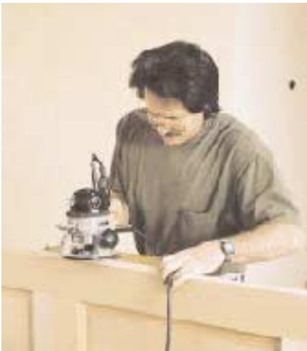
Figure 5. To mount hinges quickly and accurately, the author attaches a template over the hinge marks (top), then uses a router to cut the mortise (above left). Predrilled holes and a Vix bit speed the driving of the hinge screws (above right).
