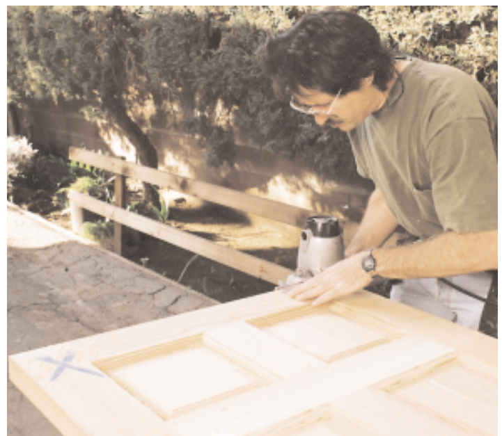
Figure 3. To ensure an even reveal at the top of the door, cut close to the scribe line with a circular saw, but finish the job with a power plane. To avoid tearout at the edges, hold the plane upside down and work the first 6 inches of the rail from one side (left), then flip the plane over and finish planing from the other side (right).
